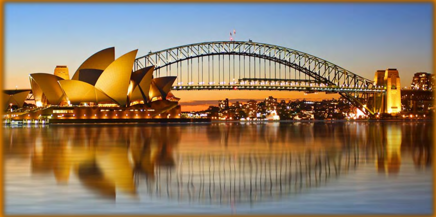
Sydney Harbour Bridge
